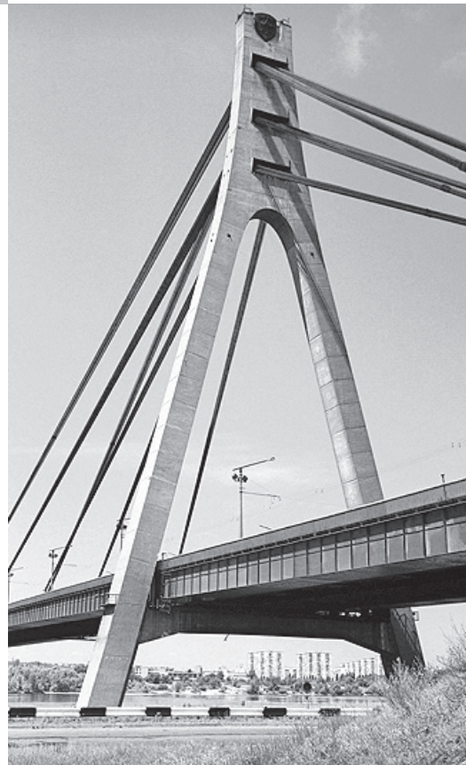
MOSCOW BRIDGE IN KIEV WAS THE FIRST LARGE CABLE-STAYED BRIDGE IN THE FORMER USSR. NOW IT'S ALREADY A HISTORY OF «MOSTOBUD»
